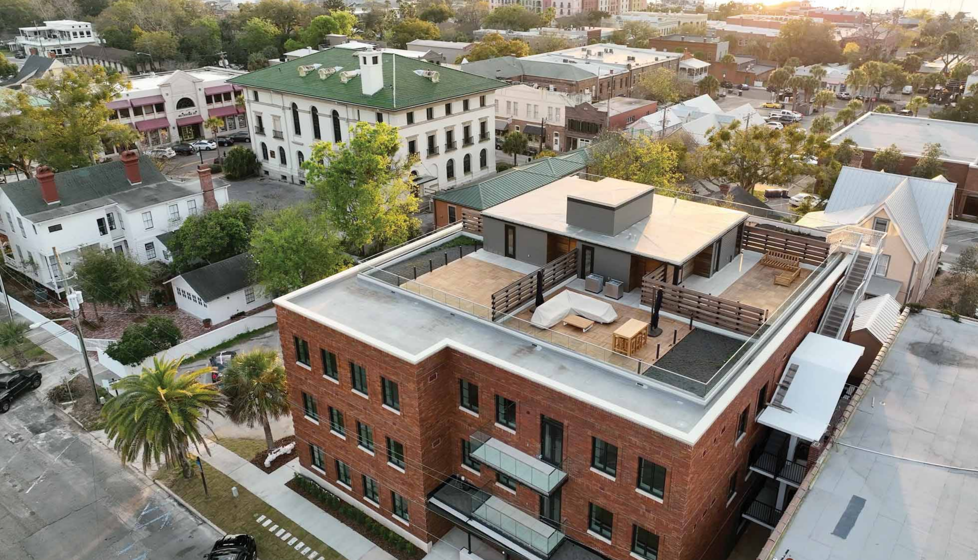
Axonometric view of the 4000 SF rooftop garden, with amenities space and four private garden terraces for 3rd floor residents
