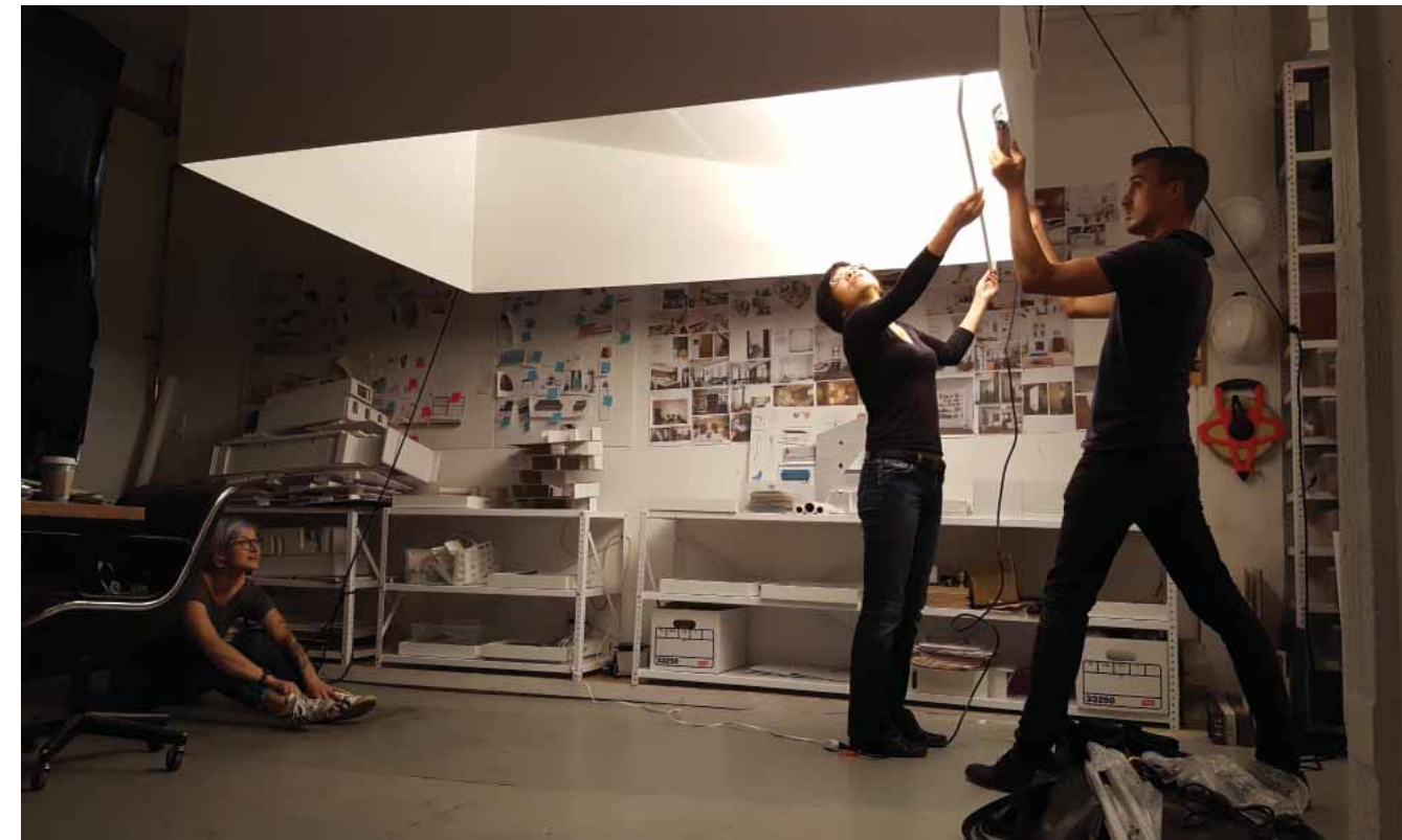
Lighting cove full-scale mock-up in studio
